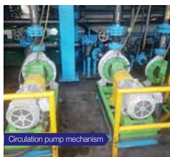
Circulation pump mechanism
