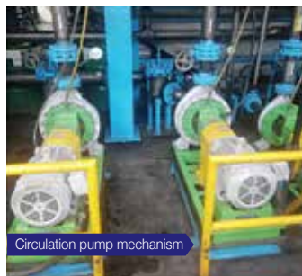
Circulation pump mechanism
